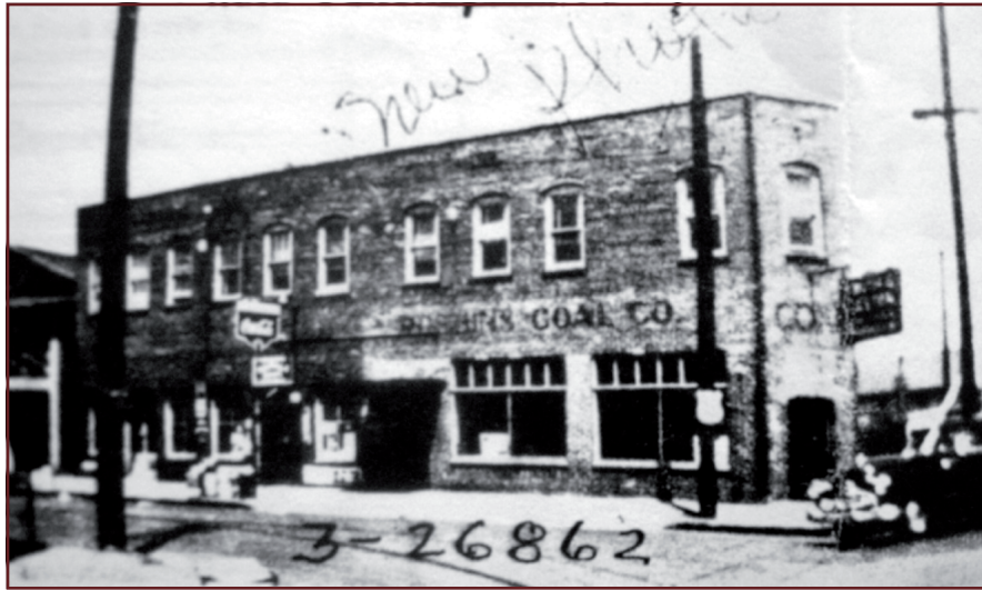
Belcher-Nixon Building, 1948 Birmingham Public Library Archives
