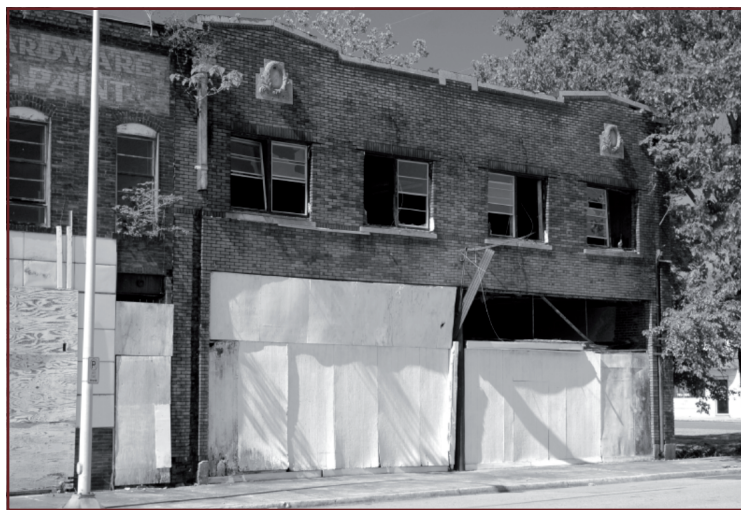
Neglected Commercial Building, 305 19th Street - Many of Ensley’s buildings are in an advancing state of deterioration.
